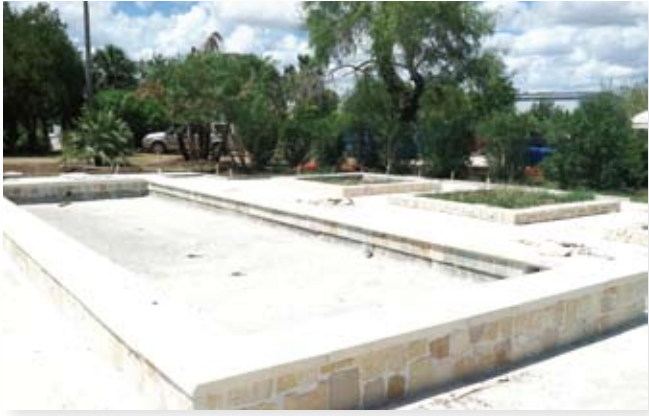
공사중인 치유 정원 Healing Garden is now under construction
